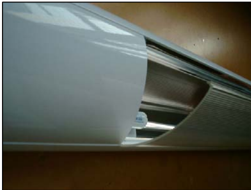
Step 1: Engage one edge full length first.
