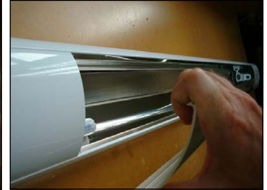
Step 4: Once started carefully tilt diffuser out using two hands to disengage full length.
